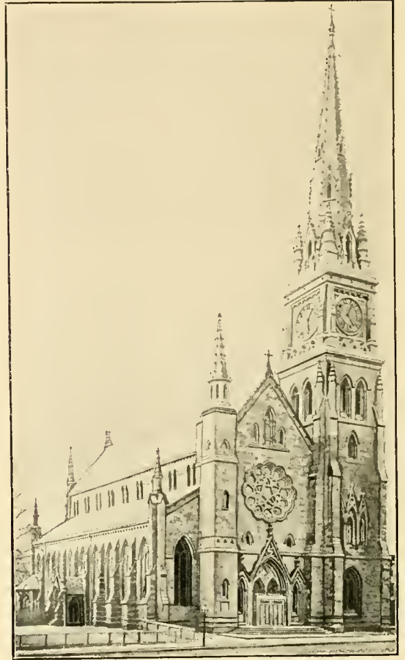
ST. JAMES' R. C. CHURCH, LAFAYETTE STREET.
